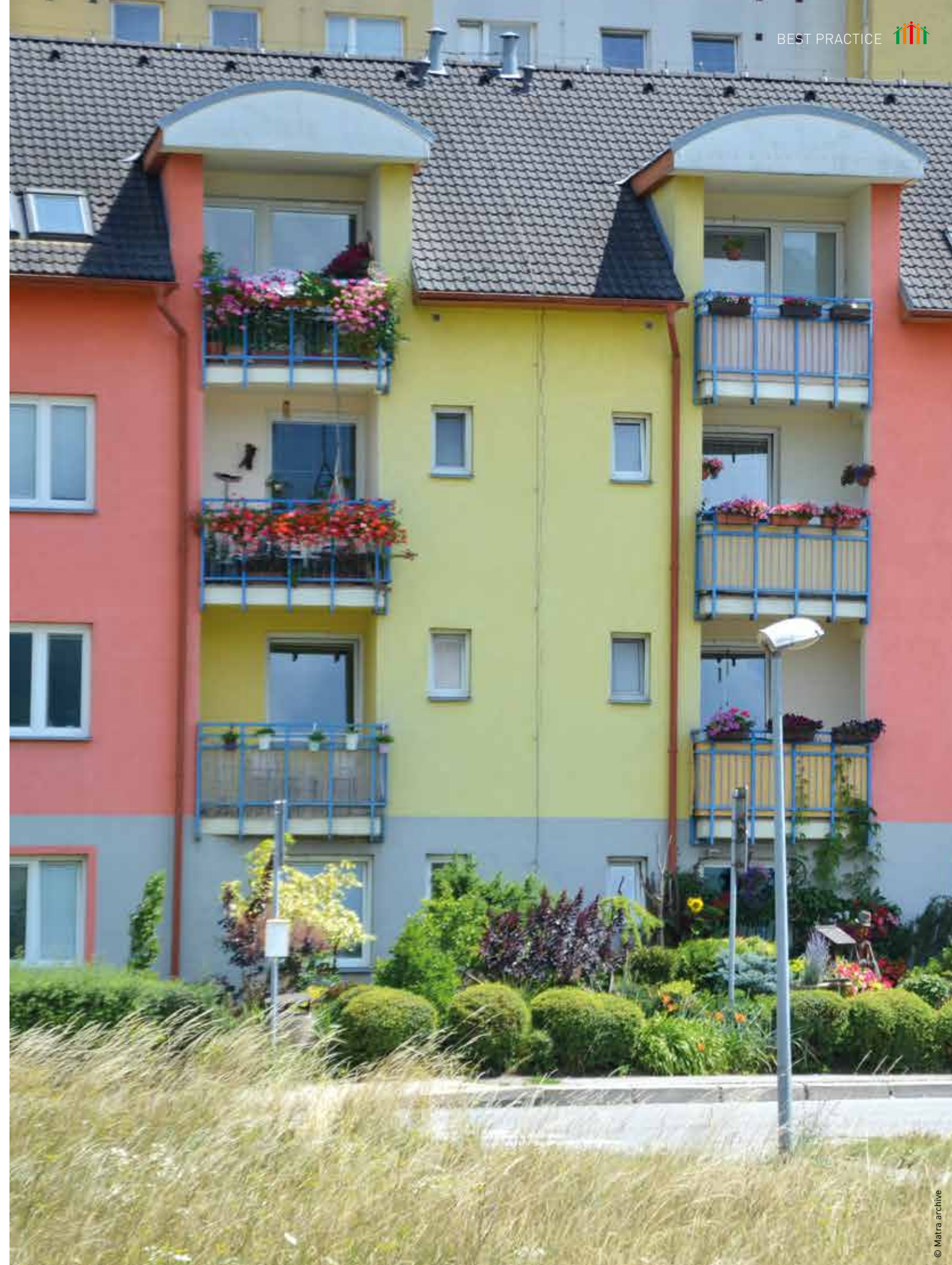
Renovated and modernised building
