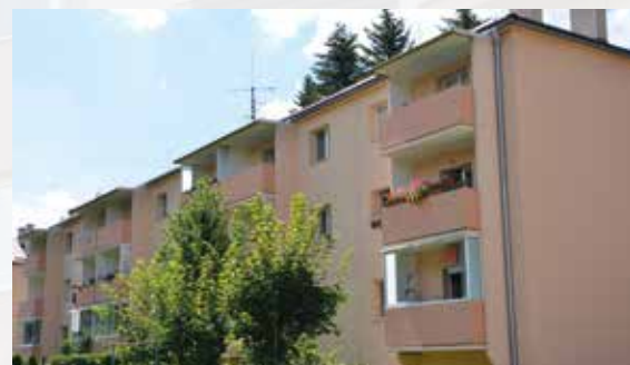
Renovated and modernised building
