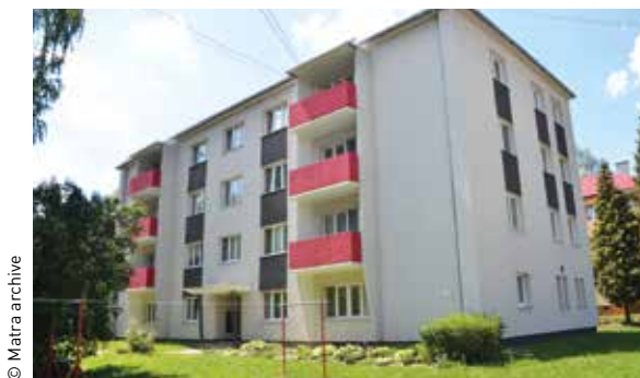
Another building of the project after renovation
